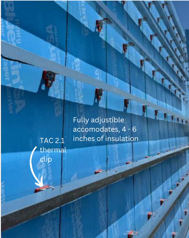
Horizontal Girt Application Accommodates 2 or 4 fasteners
