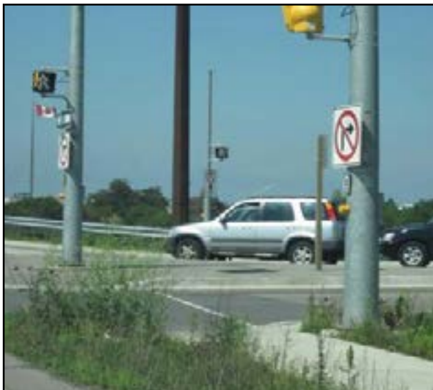
Figure 78 – Example of Municipal Sign Grouping (two regulatory signs mounted on a signal pole)
