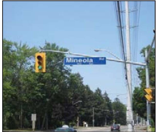
Figure 82 – Large Street Name Sign on Signal Mast Arm
