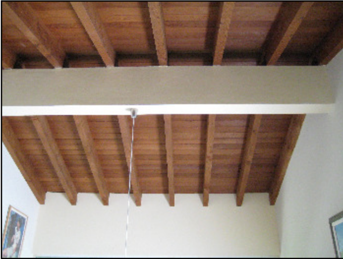
13. Rafters/roof joists
