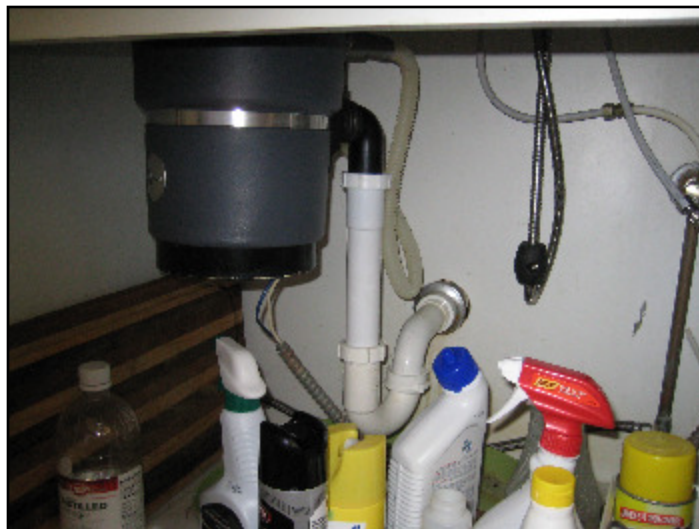
29. Loose/ Missing wire clamp
