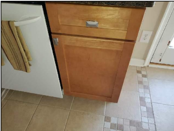
7. Doors or drawers missing or loose
