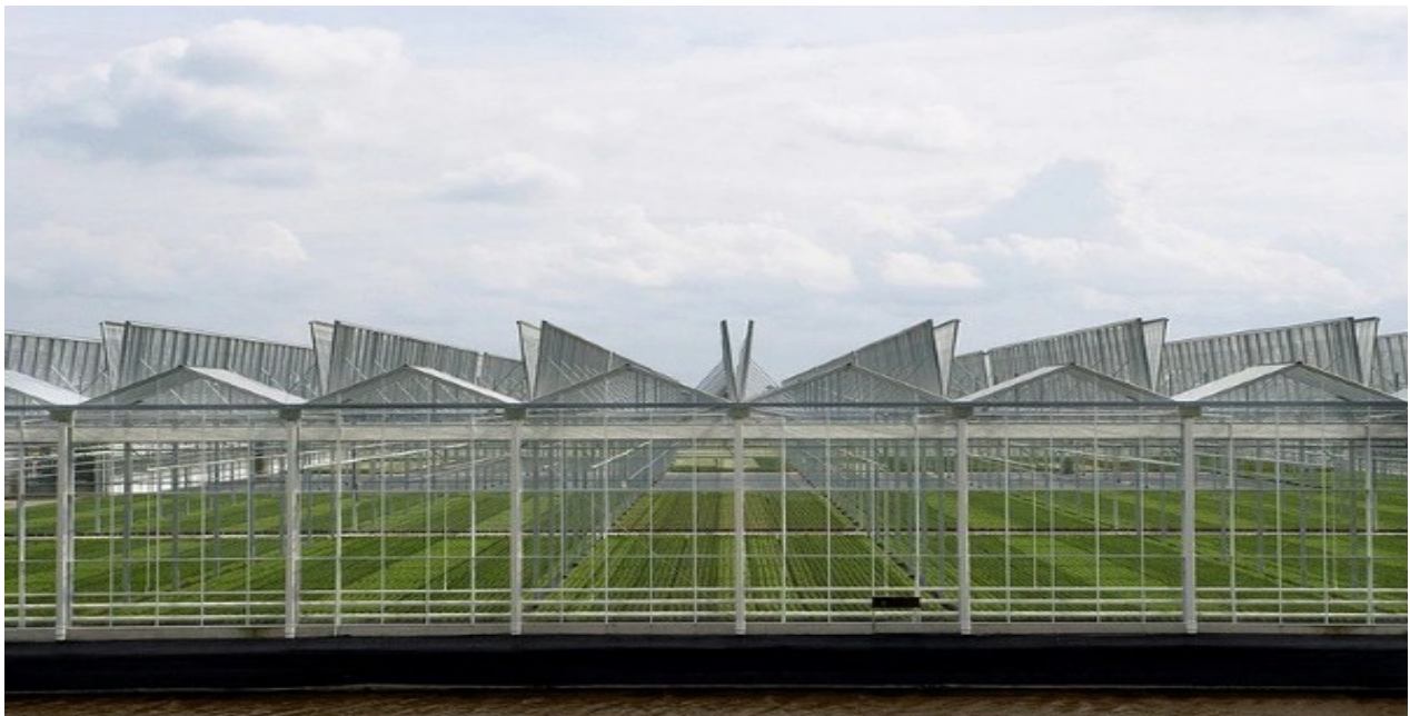
Greenhouse with open roofs to vent hot air.
