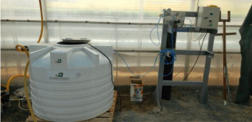
**Top left:** VCO2 system installed in a larger two hundred gallon water tank.
