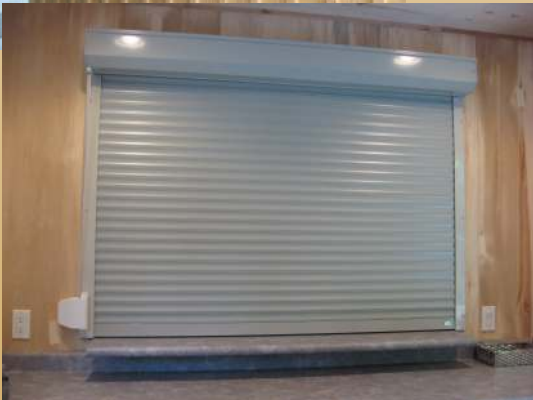
Roll shutter on Cabana, as seen from the inside
