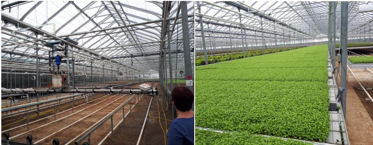
This about to be 230,000 sq ft Ontario lettuce/microgreen greenhouse is installing water spray racks over double tables of grow medium. These racks are tied into the main central water supply cross pipes (left picture centered). This grower does daily AM spraying of mostly microgreens, lettuce and basil grown in 10-30 day periods for major Ontario grocery stores.
