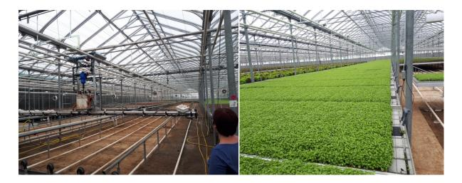
This about to be 230,000 sq. ft. Ontario lettuce/microgreen greenhouse has installed 28 water spray racks over double tables of grow medium. These racks are tied into the main central water supply cross pipes (left picture centered). This grower does mainly daily AM spraying of mostly microgreens, lettuce and basil grown in 10-30 days for major Ontario grocery stores.
