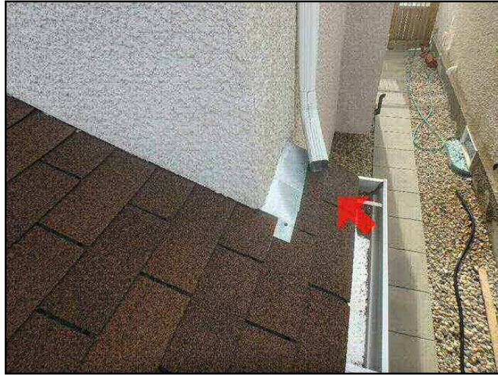
Downspouts discharging onto roofs
