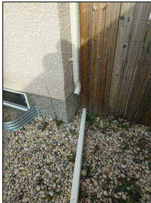
Should discharge 6 feet from building
