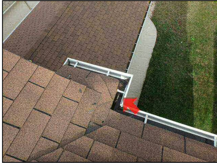
Improper slope, ponding
