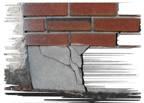
**Horizontal cracks** in foundation walls may be of most concern. They are generally found in concrete block walls, and characterized by a gap on the inside of the mortar joint only.
